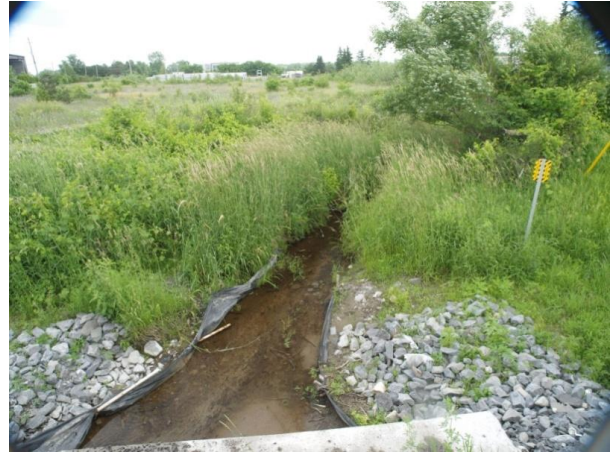
Carp Road (A) looking east at downstream end
